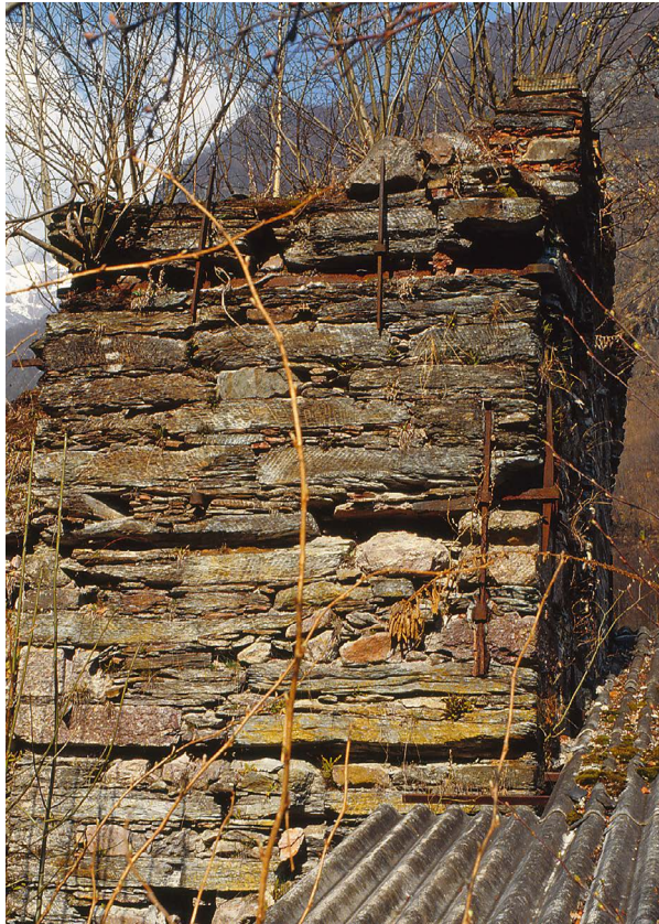
Figure 9. The remains of the blast furnace of Fiumenero (Bergamo). Photo: M. Tizzoni.
