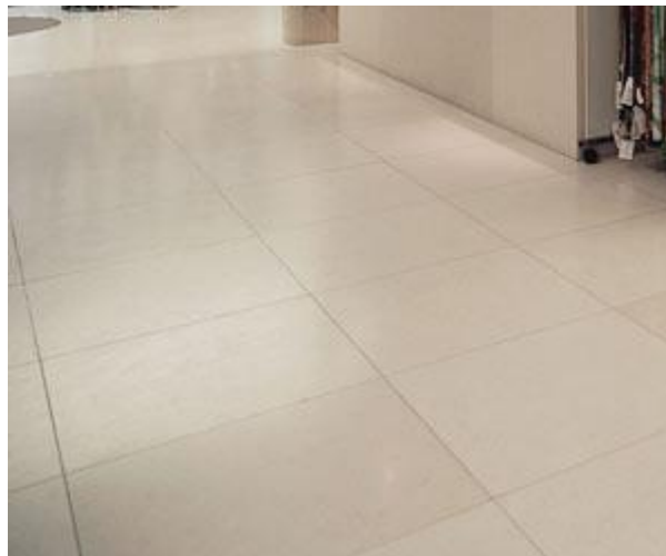
Fig. 3. An example of typical use of Moleanos limestone in flooring.
